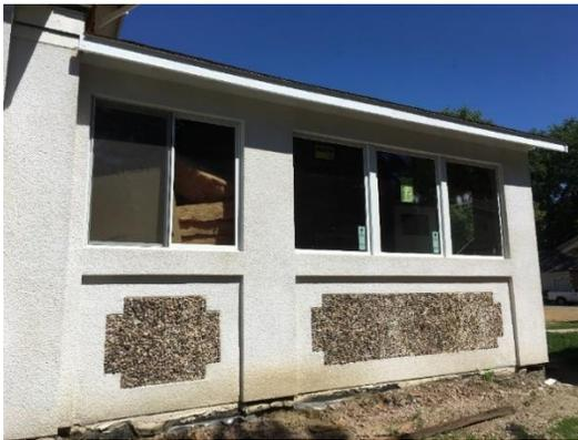
house are installed throughout. Stuccoing alone amounts to over 2000 square feet which was hand applied in three layers by master craftsmen. Only finishing details left are to install screens on the porch and painting.
